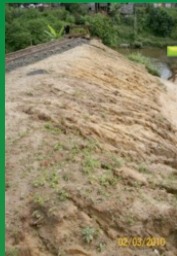
Vetiver System Application for infrastructure stabilization (railway): before/after the plantation's work
