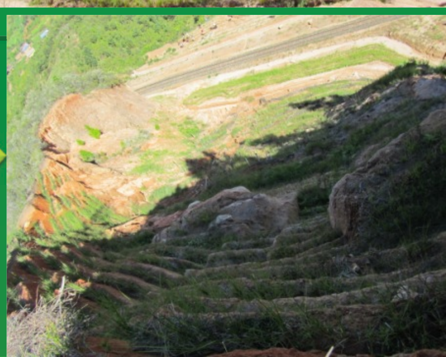
Vetiver System Application for infrastructure stabilization (railway): before/after the plantation's work
