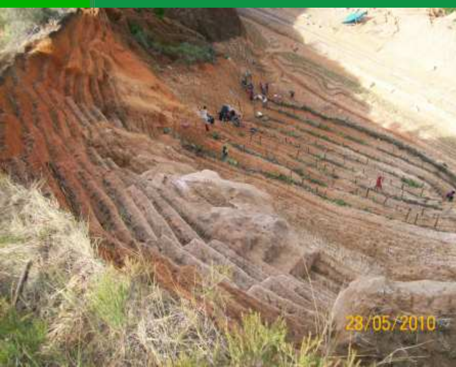
Vetiver System Application for infrastructure stabilization (railway): before/after the plantation's work
